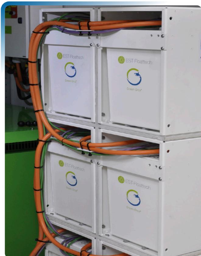
When the batteries need to be charged, the power management system signals the diesel generator. The micro grid is then run from the generator, which also charges the batteries with any spare capacity up to its at ideal engine load (80%), which is the point where you get maximum amount of power per liter of diesel. VHT provided most of the software and the technology for this system, which quickly established itself as a success.
